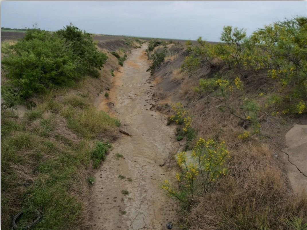
Upstream view at Station 21931
