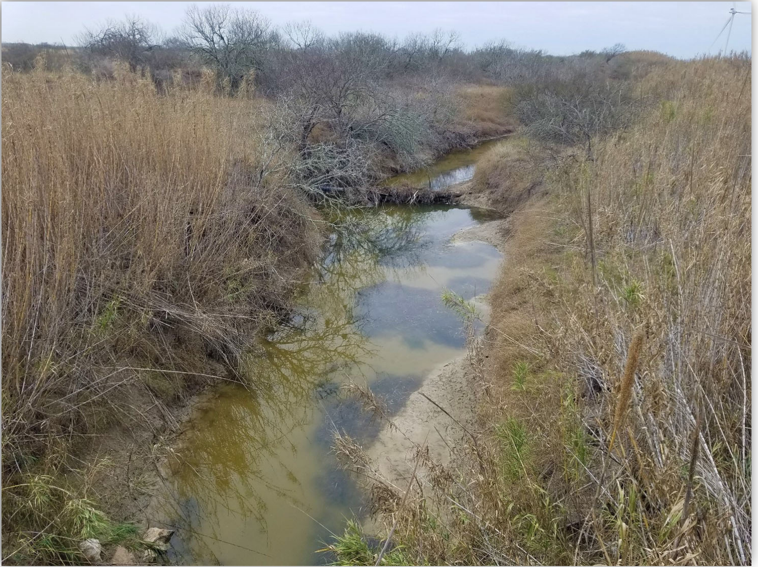
Upstream view at Station 18642
