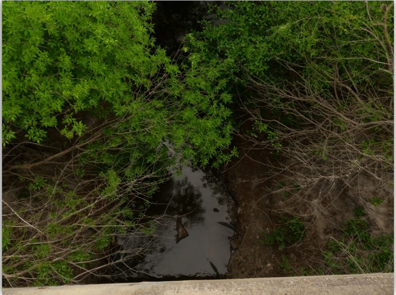
Upstream view at Station 13094
