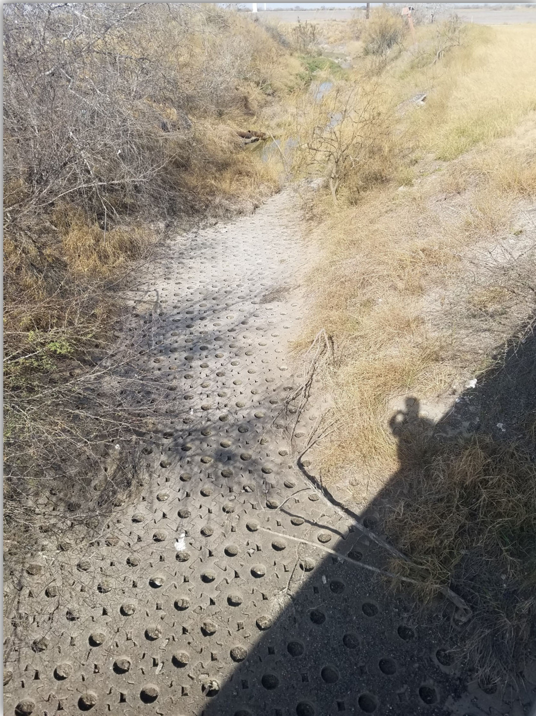
Upstream view at Station 21596
