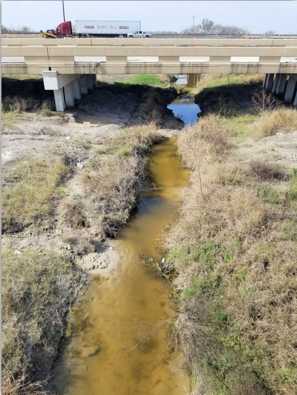
Upstream view at Station 21594
