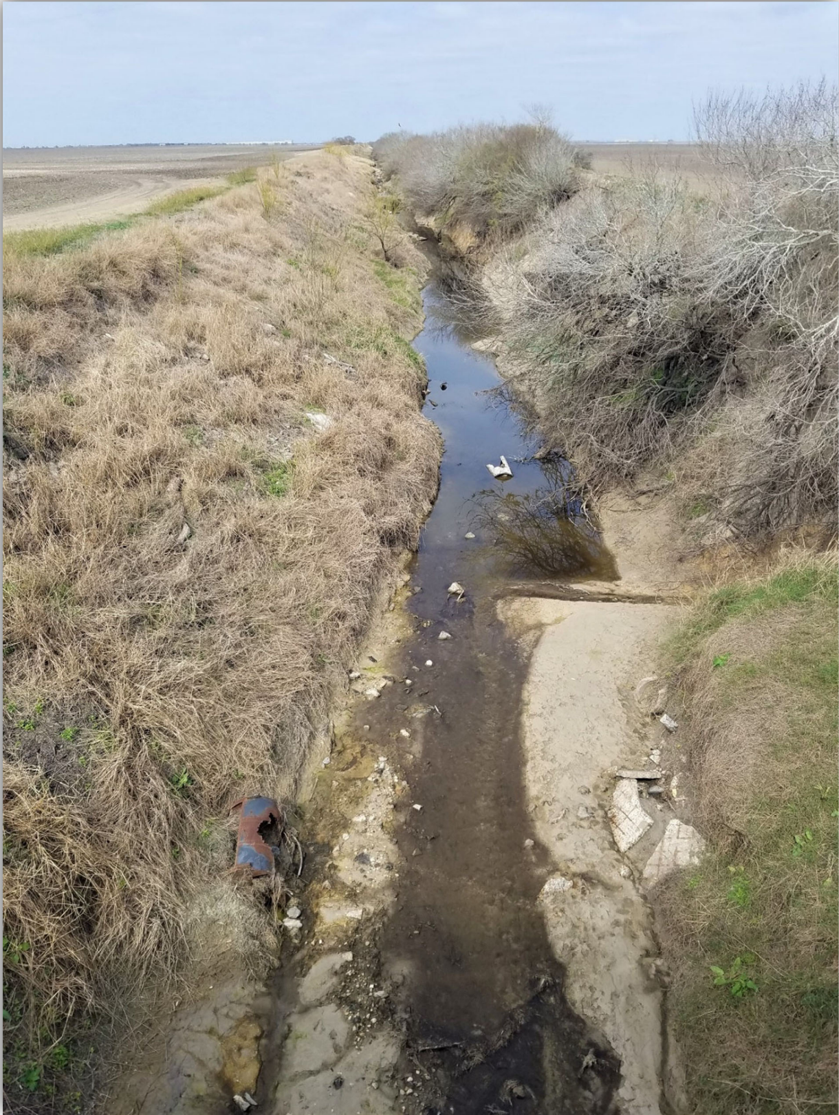
Upstream view at Station 18484
