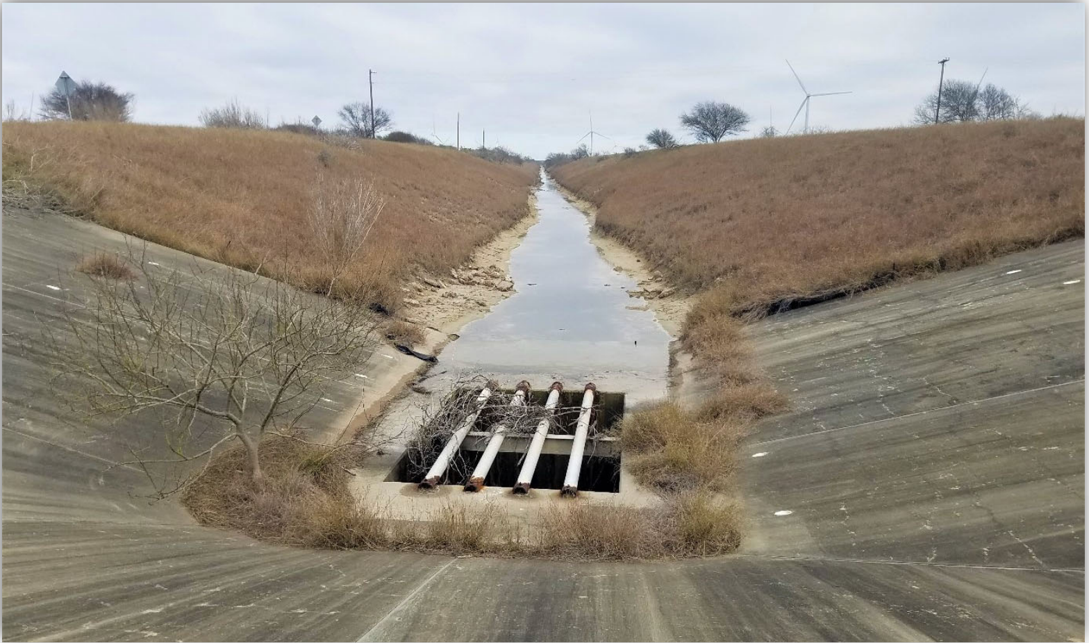
Upstream view at Station 21928
