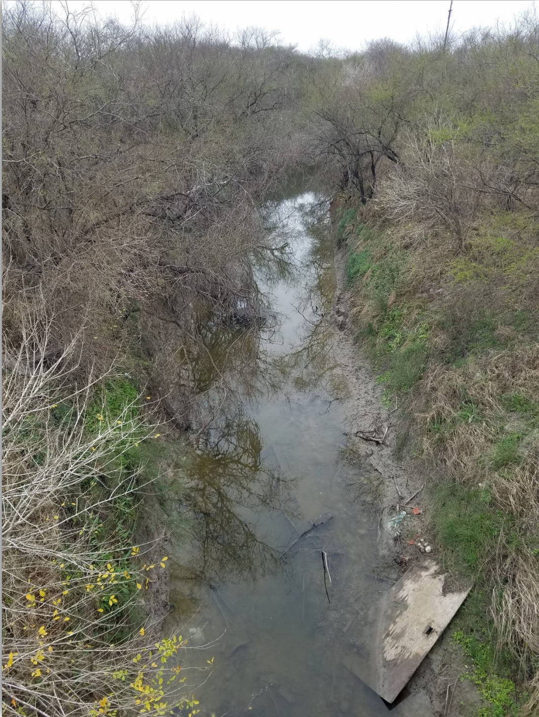
Upstream view at Station 13095
