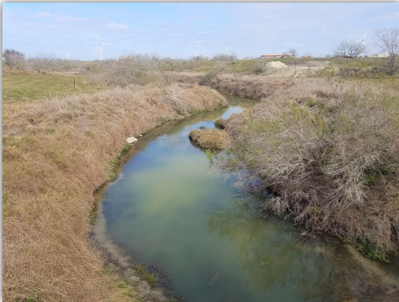
Upstream view at Station 13030
