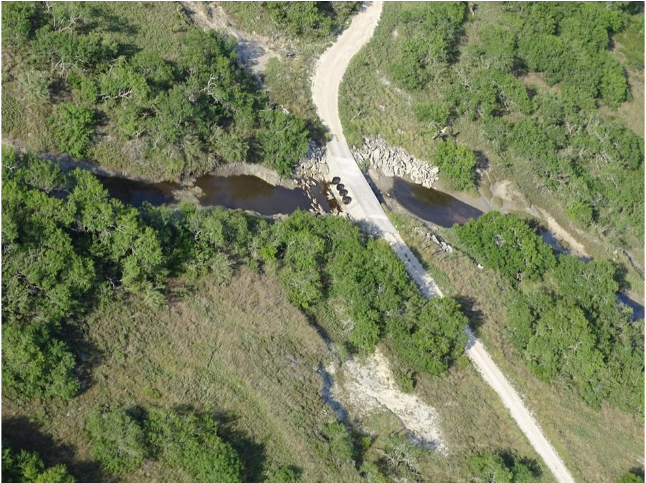
Figure 37 This image shows a poorly designed crossing on Jaboncillos Creek. It appears that the creek has down cut around the crossing and left its conduits high and dry. Piles of cement debris can be seen dumped along the channel around the crossing in an apparent attempt to dissipate stream energy. Stream crossings should always be located on a straight section of channel to avoid excessive stream energy being directed at the crossing.
