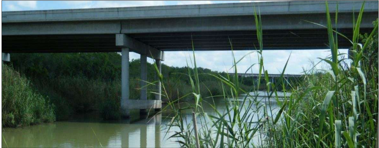
Figure 3: Arroyo Colorado at Cemetery Road
