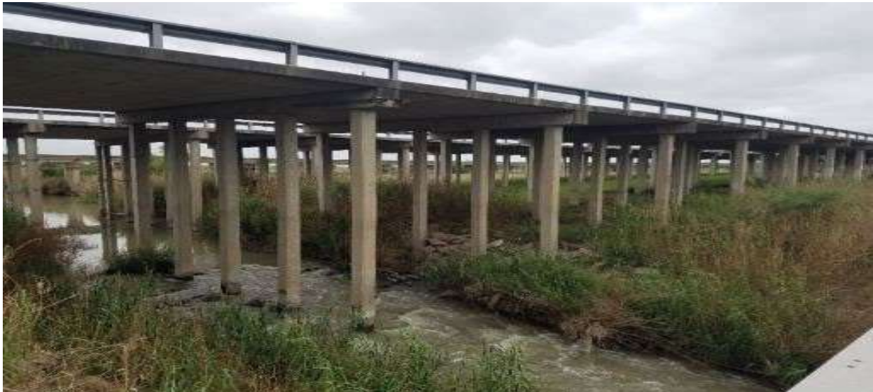
Figure 34: North Floodway Station 20930
