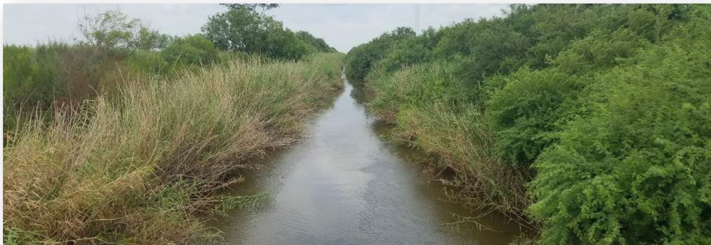
Station 22003 – Raymondville Drain at CR 445
