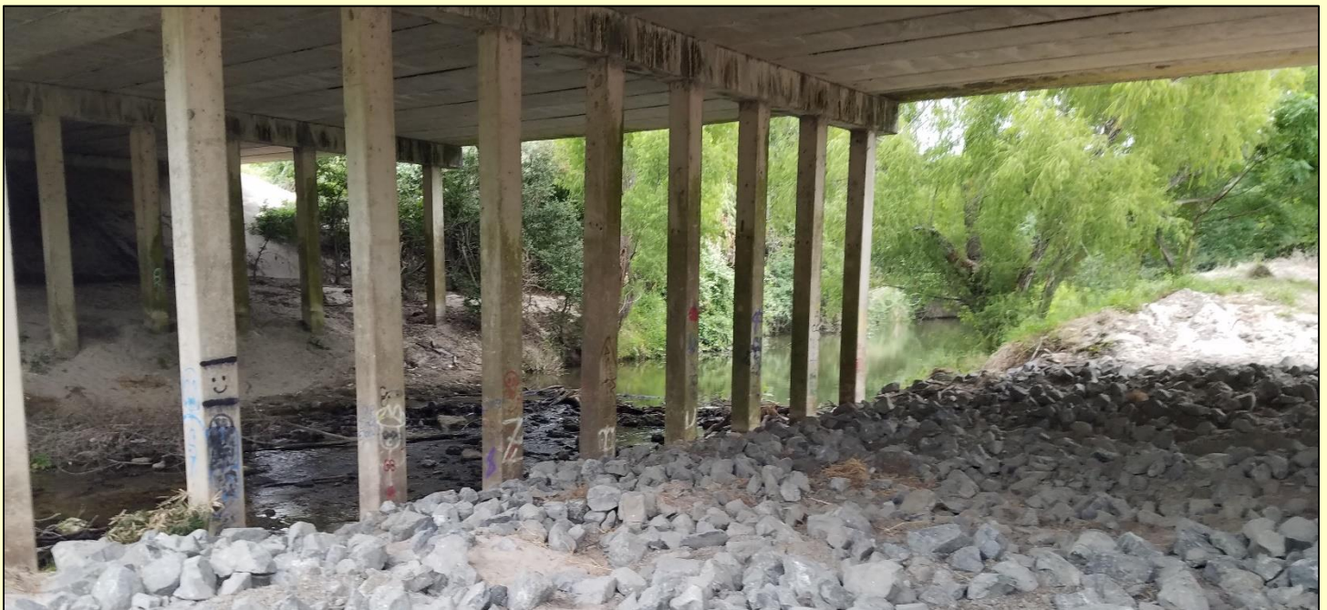
Station 12937 – Erosion Control at Poesta Creek at FM 202 near Beeville on June 15 th , 2022
