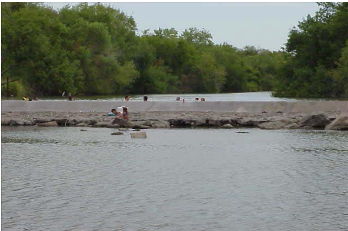
Figure 2. Photograph of the Calallen Saltwater Barrier Dam.
