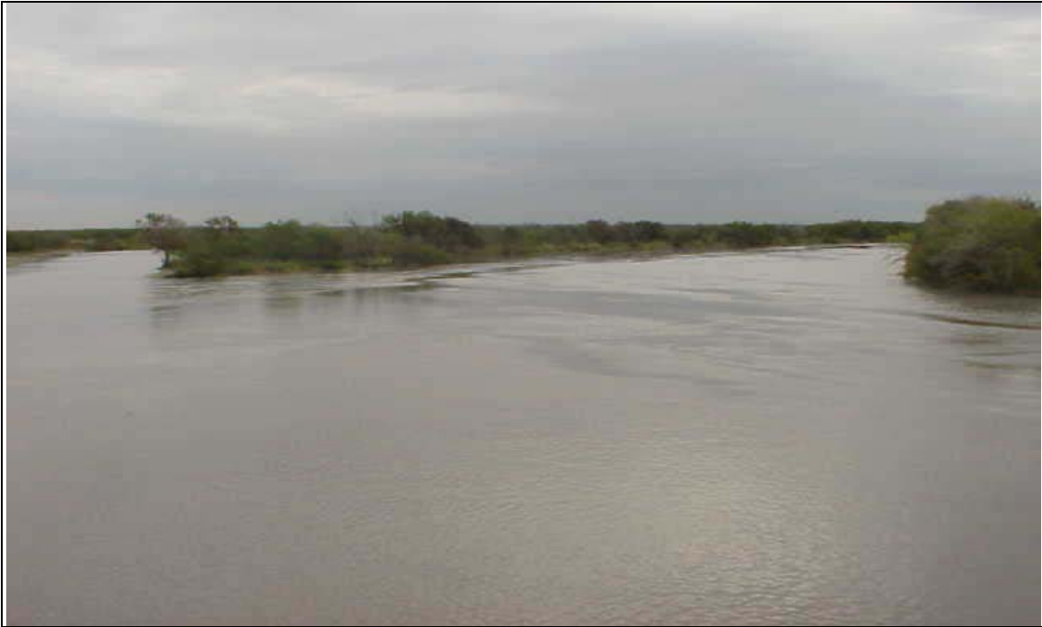
Figure 3. View from IH-37 Bridge overlooking site 12961 and Nueces Overflow Channel during high flow conditions.
